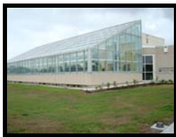
The quarantine facility at the USDA-ARS Invasive Plant Research Laboratory in Ft. Lauderdale, Florida
